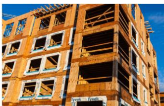
fig (6) Wood-framed apartment construction in Vancouver, Canada [3]
