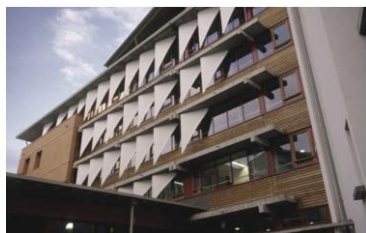
Fig (29) Seven-story office building in Clermont Ferrand which uses hemp lime blocks, and hempcrete panels as shading units on the façade. (Rachel, Tom, 2008)
