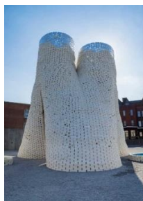
Fig (48) The 13-m-tall tower in Benjamin -New York is made of corn stalks . [50]
