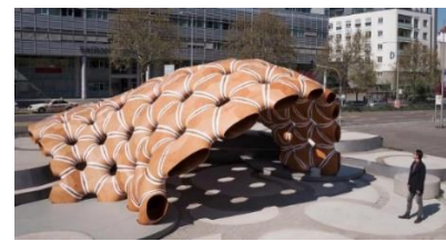
fig (17) Robots build sea urchin prefab pavilion using biomimicry [17]
