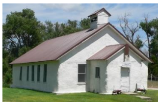
fig (35) The first rice straw building, Nebraska (bearing load system [38].
