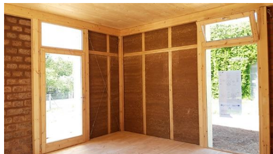
Fig (49) A prototype construction from corn and sunflower stalks by Valles school of architecture. [51]
