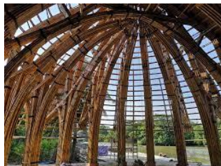
fig (19) Thailand-pavilion-bamboo build
