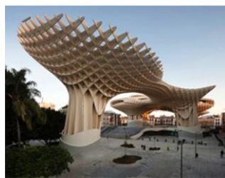
fig (16) Metropol Parasol Structure [16]
