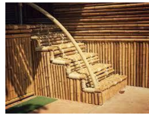
fig (20) Bamboo is used as stairs material
