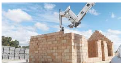
Fig (39) The usage of robots in the uniform building of bearing walls from straw blocks.
