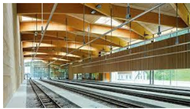
fig (8 a) Large span beams
