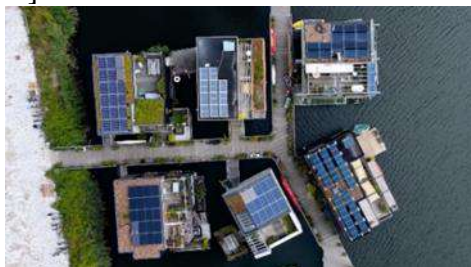
figure 12 roof-top solar collectors [9]
