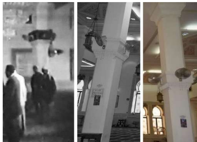
Figure 10 Al Othman Mosque columns (Al Othman Trust & the Author)
