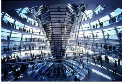
Figure (16) shows the conical mirror used to get rid of hot air and reflect the sun's rays
