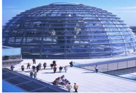
Figure (17) shows an external image of the glass dome connected between the internal and external environment by means of the advanced building technology
