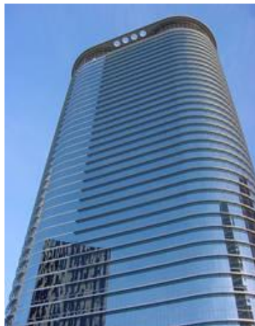
Figure (25) using self-cleaning glass
