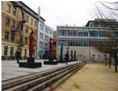
Figure: Relationship between old factory buildings and newly extended buildings. (WANG Jianguo, JIANG Nan,2007).
