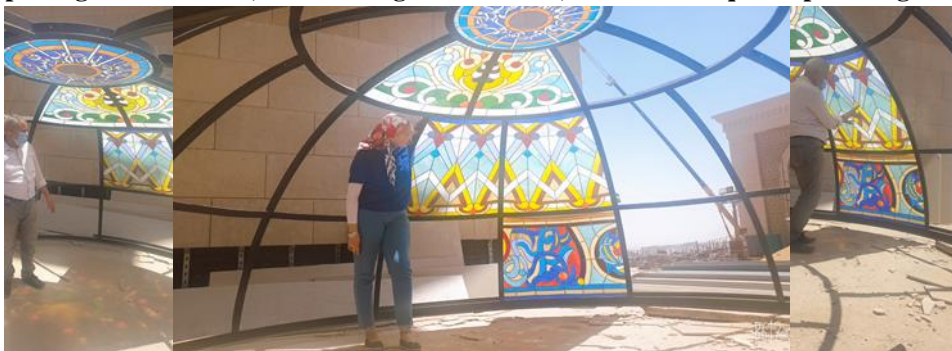
Shape 28 clarifies the experiment of first lobe of dovetailed glass on metal constructional sectors related to the dome
