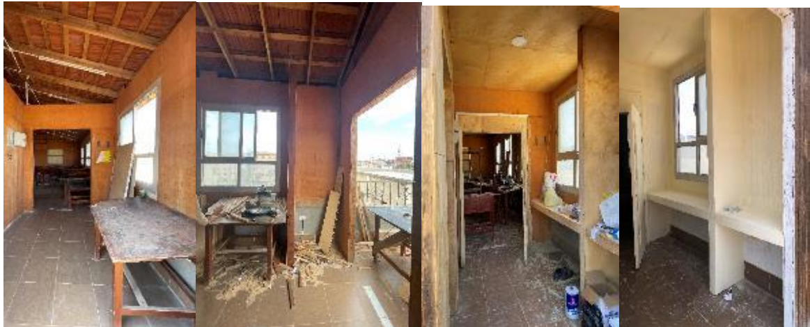
Photos n. (26) show the wall GG` before, though, and after implementation.
