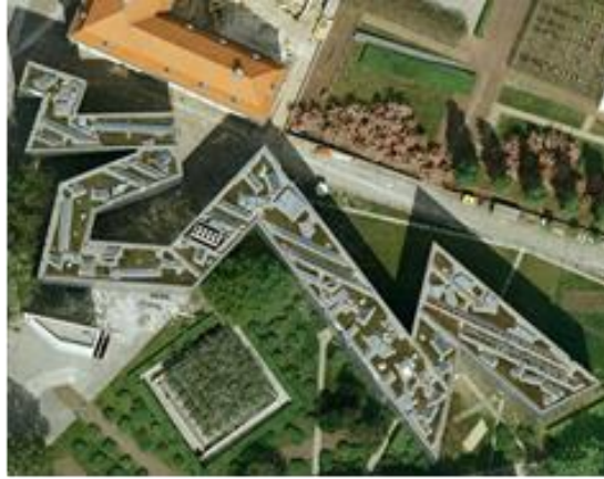
Fig.4- The general site shows the Zigzag formation of the Jewish Museum's blocks Source: Satellite Snapshot through Google Earth
