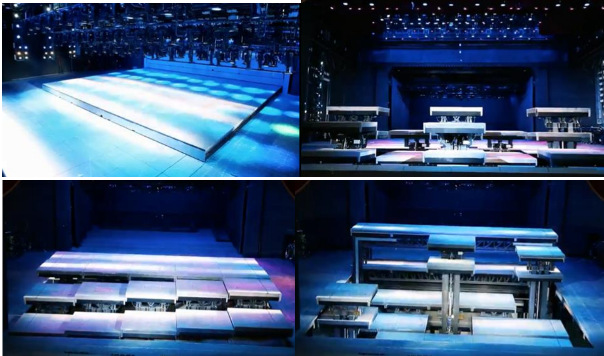
Fig 17, the stage elevator systems
