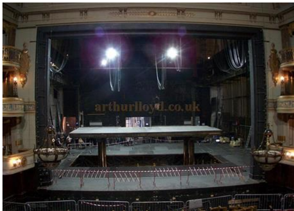
Fig 2 Each bridge is 40 feet long and 6 feet wide. To form an area of 240 feet that can be vertically heightened by 8 feet, in addition to the possibility of moving each bridge independently, providing complete flexibility, and one of the parts of the bridge can be tilted from the other part to serve the dramatic event on the stage.
