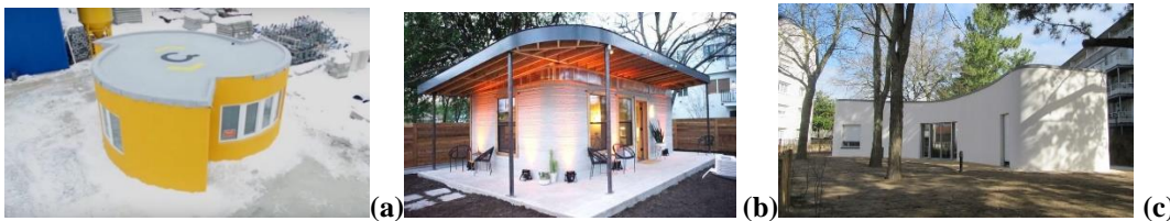
Figure 2. The faster and low cost 3D printed houses around the world (a) Apis Cor 3D printed house, in just 24 hours with $10,000, Russia. (b) ICON & New Story 3D printed house in 24 hours, with cost of $10,000, USA. (c) The First family move into a 3D printed house in France, with almost price of: $170,000, in 54 hours (Carolo 2020; 3dsourced 2021).
