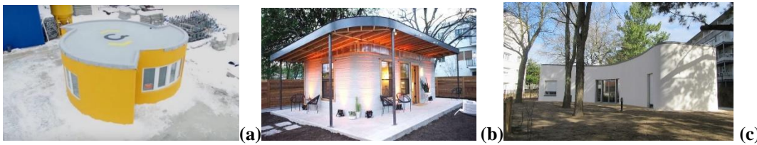
Figure 2. The faster and low cost 3D printed houses around the world (a) Apis Cor 3D printed house, in just 24 hours with $10,000, Russia. (b) ICON & New Story 3D printed house in 24 hours, with cost of $10,000, USA. (c) The First family move into a 3D printed house in France, with almost price of: $170,000, in 54 hours (Carolo 2020; 3dsourced 2021).
