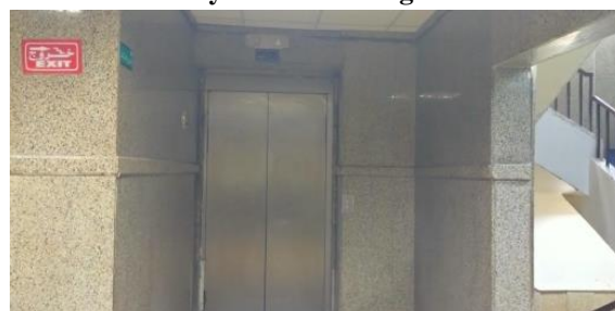
Figure (36) A field photo of the researcher showing the elevator lobby.
