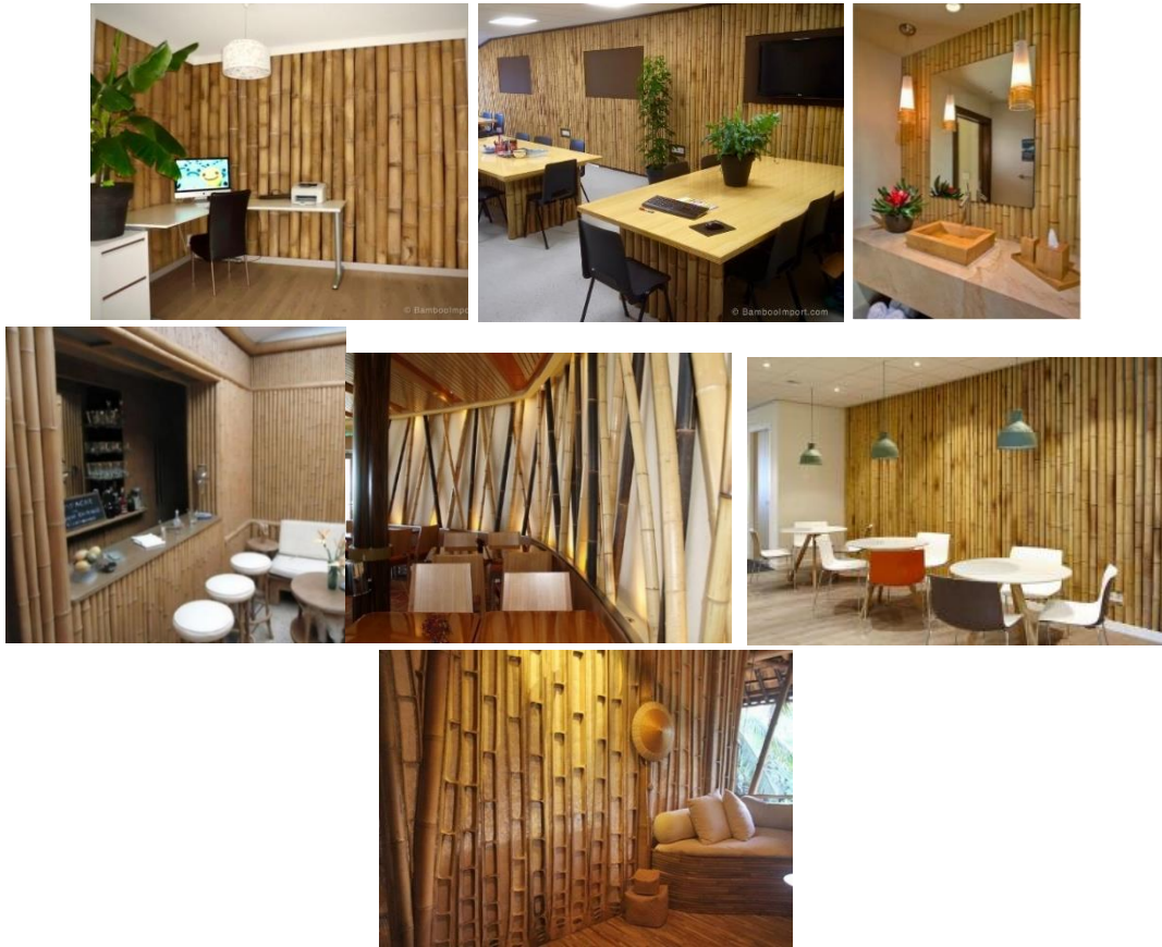
(Figure 8) Using whole or halved bamboo sheet in interior wall of different spaces.
