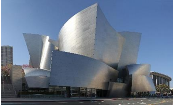
FIGURE 17. WALT DISNEY CONCERT HALL (WDCH), LOS ANGELES, CALIFORNIA
