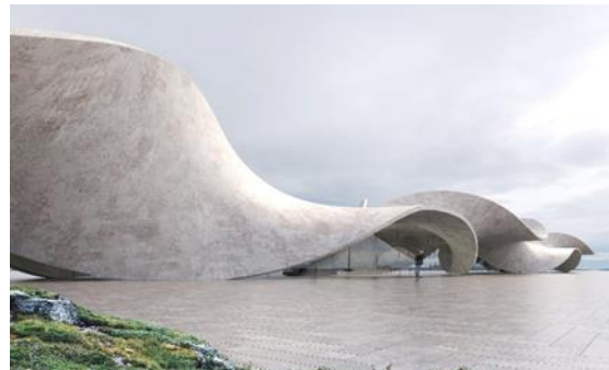
FIGURE 20. THE TWISTED SCULPTURE-LIKE CONCRETE HOUSE BY ANTONY GIBBON, ALIGNED THROUGH THE LANDSCAPE
