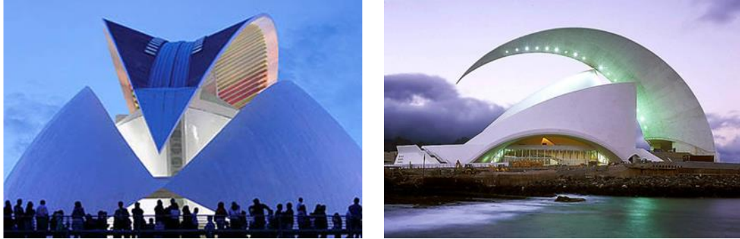
Fig.19- Opera Tenerife, Santa Cruz de Tenerife, Spain. Santiago Calatrava, 2003
