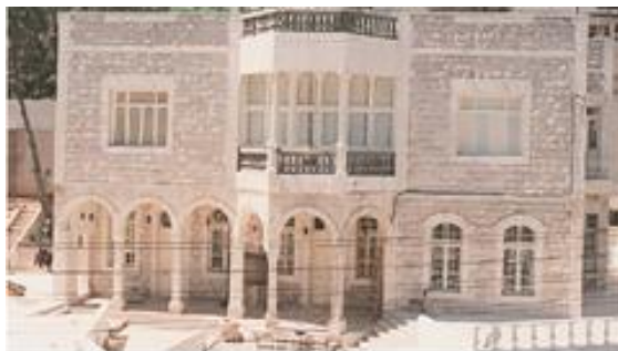
Photo (1) The Jordanian Art House by Fawaz al-Muhanna, showing the preservation of the local identity of the place through the use of arches influenced by Ottoman architecture, and some stone details at the openings
