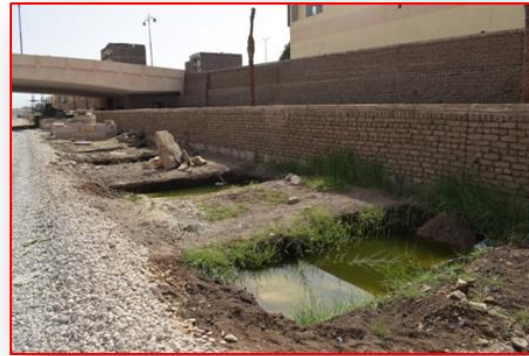
Fig (5). The presence of ground water in the site
