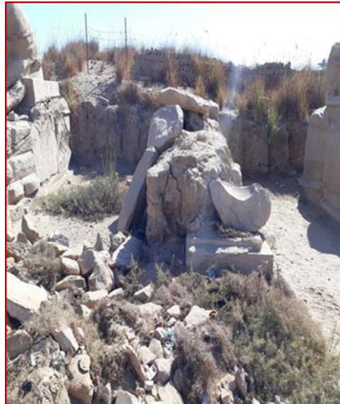
Fig (7). The condition of some of the bases of the road, which are destroyed and weeds spread, and the presence of cracks and many separations is noted
