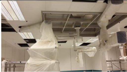
Figure (1-11): The air unit above the patient's bed, laminar air flow, at the Neuroscience Center at King Abdullah Medical City in Makkah
