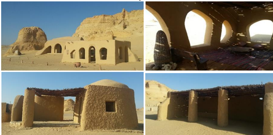
Fig. 12: The cafeteria, Visitors Centre and gift shop at the Wadi Al-Hitan National Park. Mud brick, reed, and plaster as building materials deeply entwines in the regions culture. Photos taken by the Author.
