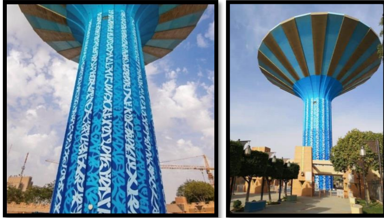
(Figure 2) Water Tower - Riyadh - Kingdom of Saudi Arabia – 2019
