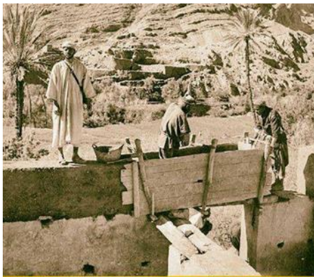
Fig. (29): Construction of walls by Tapia, https://www.facebook.com/dakirati_znit/
