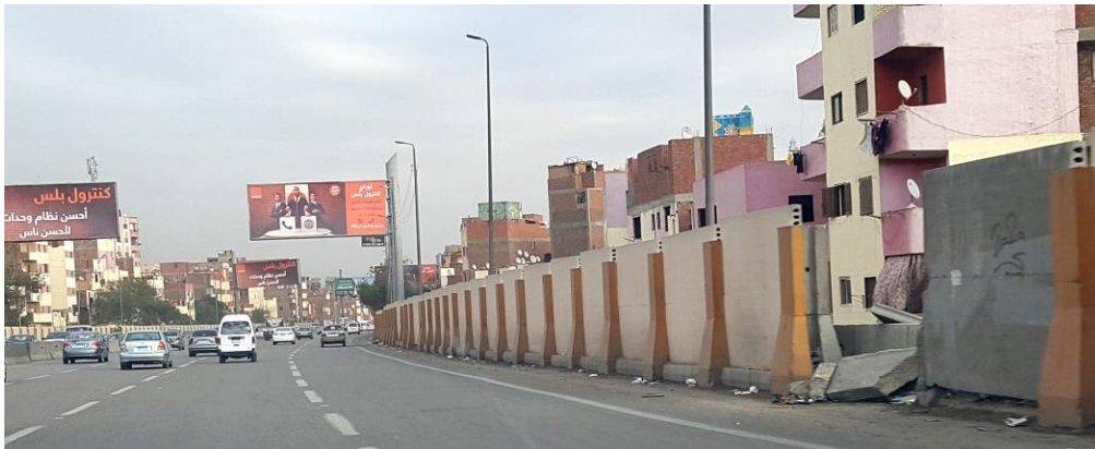
(Figure 11) The fence executed on the ring, which distorts the facade.
