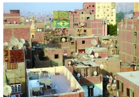
Figure 8. Neglect and non-exploitation of residential roofs
