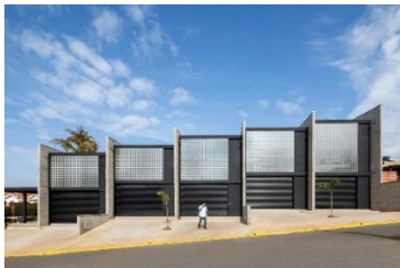
FIGURE 46. CL WAREHOUSES / VAGA https://www.archdaily.com/926816/cl-warehouses-vaga Accessed 16 Nov 2020.
