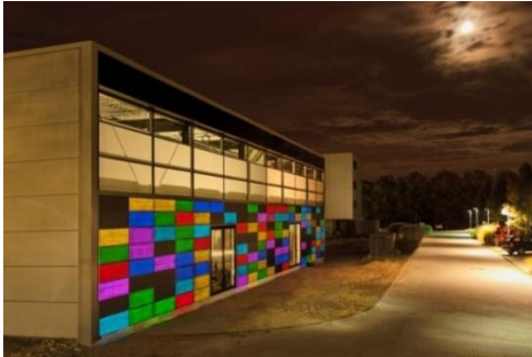
“Using light-transmitting concrete in exterior facades and interior design works, showing the possibility of using colored lights on them”.
