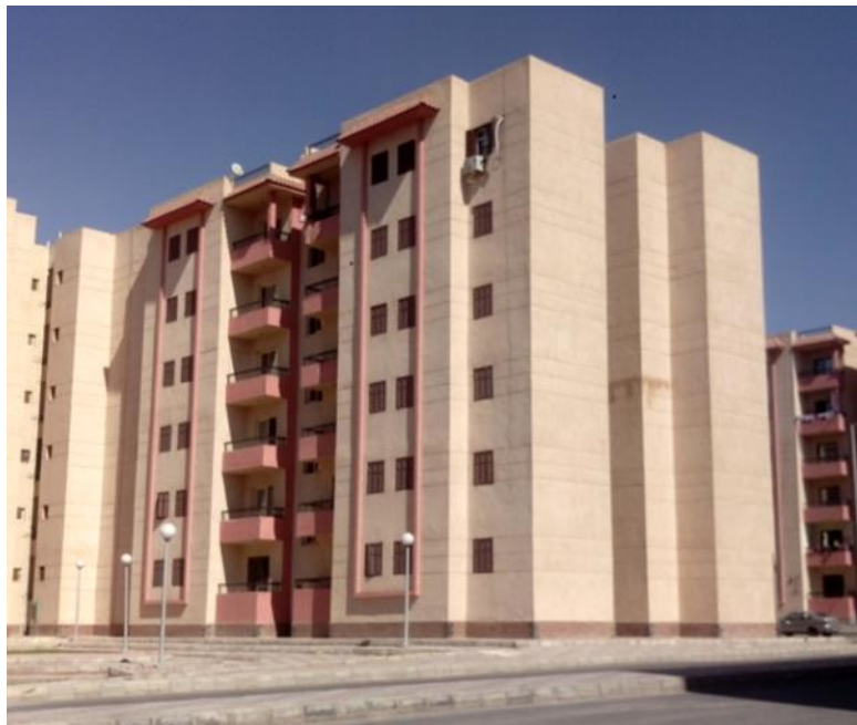
Figure (3) shows a model of a residential building - social housing of 800 acres - New 6 th of October City - Giza.
