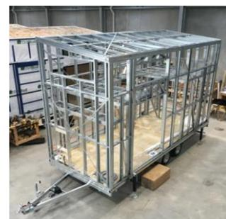
FIG.1: THE CHASSIS OF THE GALVANIZED STEEL LIVING STRUCTURE AND THE SECTOR USED FOR STRUCTURE.
