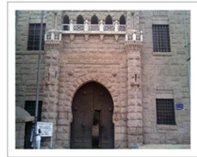
fig. (1) the main entrance
