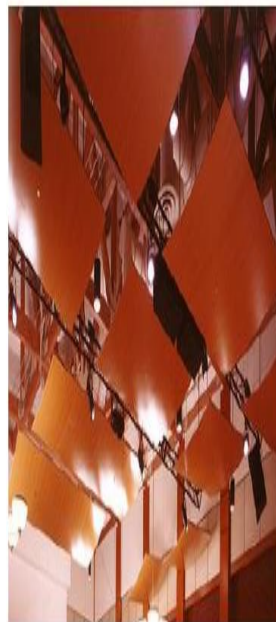
Figure (13) shows Reflector Panels that are scattering sound waves in different
