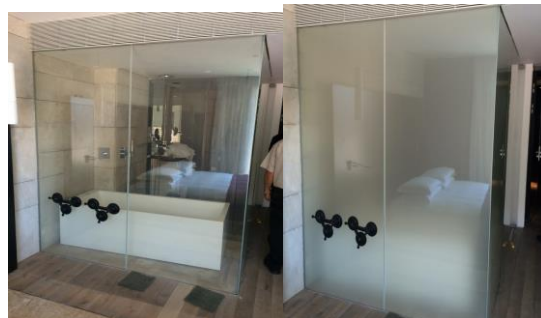
Figure (2) shows the use of chromo electric materials in the interior glass breaks.
