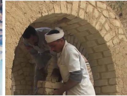
Fig.8&9 Hauf-Rif (Morocco) regular and irregular Implementation of mud brick installed, mortar and brick are from the same material.
