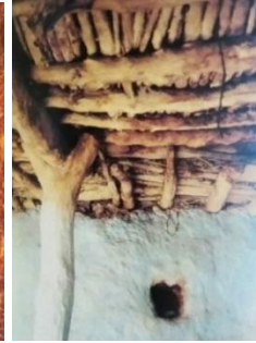
Fig.7 Haut (Morocco) The masonry took advantage of the natural tree shape with a trunk to support the trunks above.
