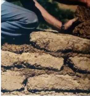
Fig.6 Ghardaia Village (Algeria) - The accuracy of the solid lime stone slabs closure, with extended beams of palm trunks.
