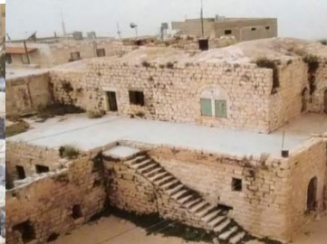
Fig.3 Aures ( Algeria) An unfamiliar construction, wood is used with stone to improve the performance of the wall structure - these fixing systems provide the opportunity to use irregular stones linking the two surfaces to increase stability, bonding and to resist earthquakes without disturbing the building balance.
