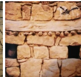
Fig.4 Irbid (Jordan) - Ashlar stone masonry construction is cut with saw or chisel which is of 4, 5 or 6 faces - The construction is made of limestone and basalt layers, the surface is engraved.
