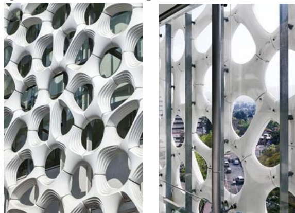
Fig (12) The shape of the envelope surrounding the building from an external and internal perspective
