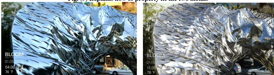
Fig. (10) Demonstrates the mechanical movement caused by bimetallic thermal materials with varying temperatures at the Bloom Gallery in Los Angeles
