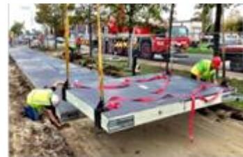
Figure (21): Modules of silicon crystalline solar cells, which are combined with a concrete layer.
