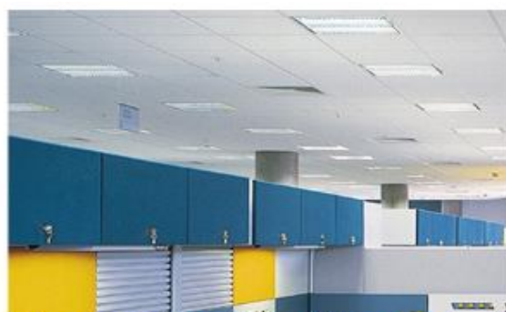
Picture No. (12) shows the use of the gypsum board tiles in the ceilings of the administrative area of the Psychiatric Hospital: https://www.usgboral.com
