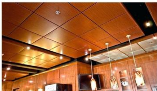
Picture No. (13). shows the use of soundproof ceiling tiles in a psychiatric hospital reception area / : http://makanankhas.xyz/edit
