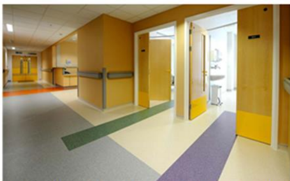
Picture No. (7) shows the use of vinyl panels on the walls of psychiatric hospitals
