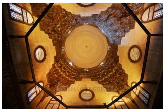
Figure 23 b: The four corners with four fractal muqarnas shapes.
