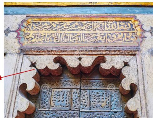
Figure 22b: the top of the door.
