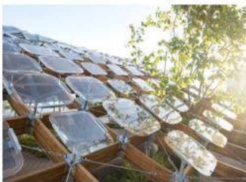
Picture of corrugated roof over open mesh structure and the use of electric power panels.
