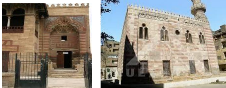
pic Nos. (4 and 5) indicates the entrance and backside of Sultan Qaytbay School Reported by
