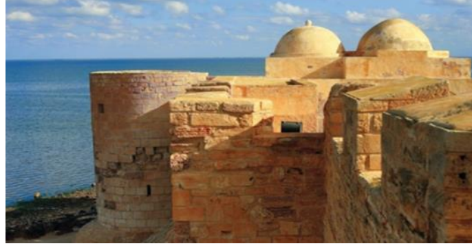
Pic No. (44) indicates Tagdet Mosque in Tunisian Djerba island, Fatou area in the north of the island
