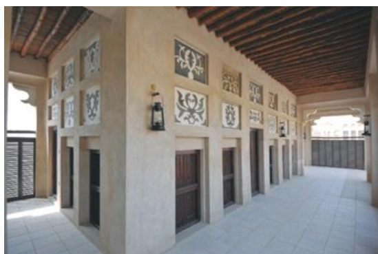
Shape 17 shows ornamented claddings
