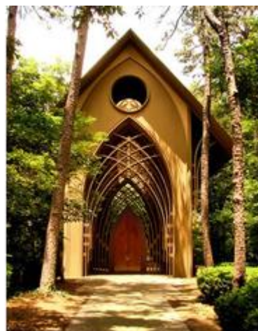
(Fig. 3) the church from the outside http://beautifulbellavista.com/chapel.htm
