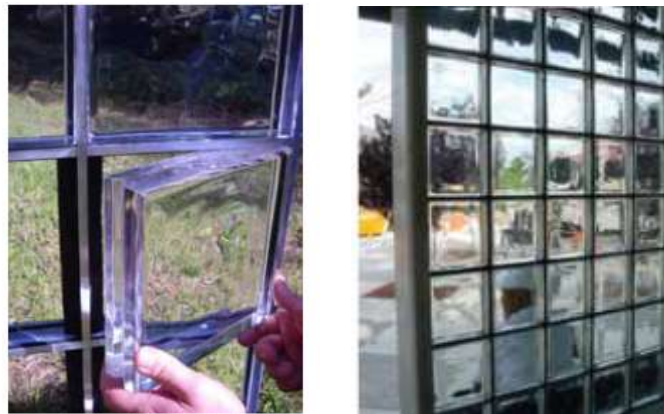
Figure (5) shows the method of installing blocks inside the aluminum sections
