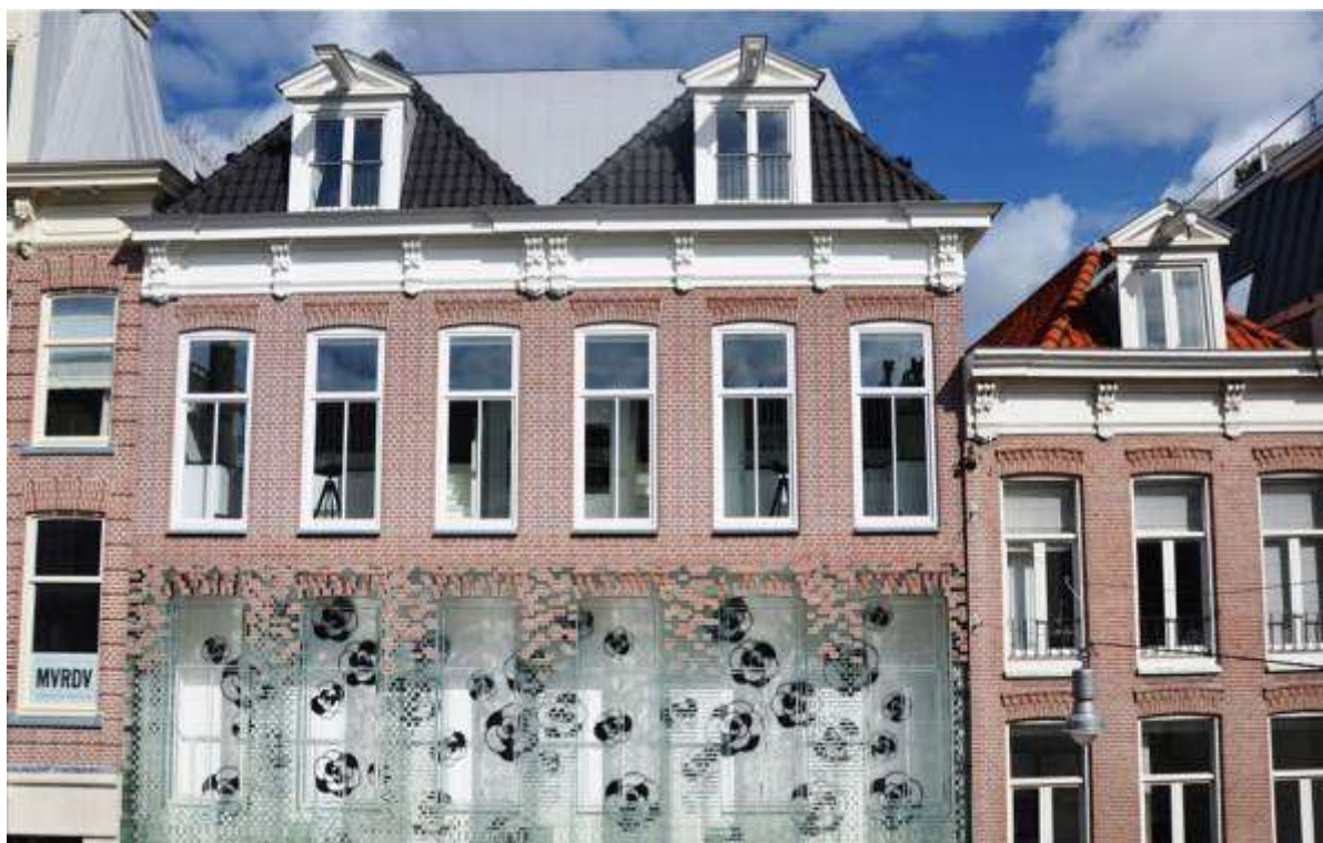
Figure (7) shows the image of the building after the final installation of the wall made of glass blocks
