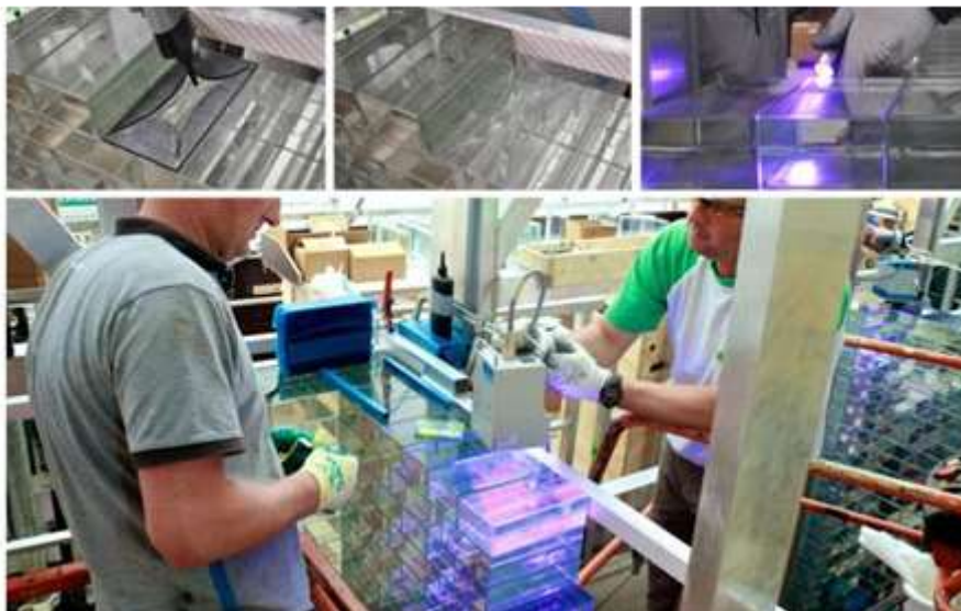
FIGURE (6) illustrates the method of gluing between blocks and reinforcing them with UV radiation
