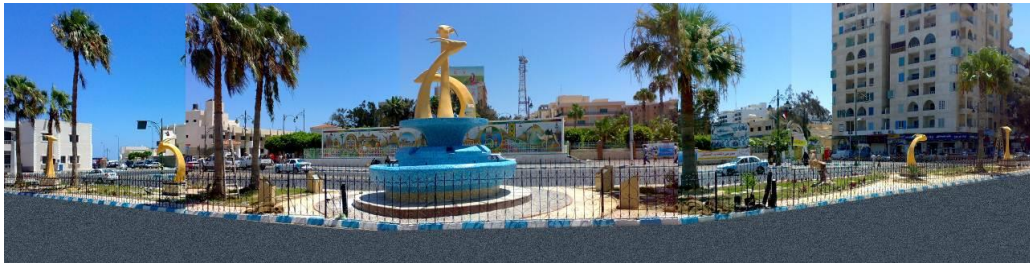
Details from the refuge island at Matrouh governorate after finishing the project.
