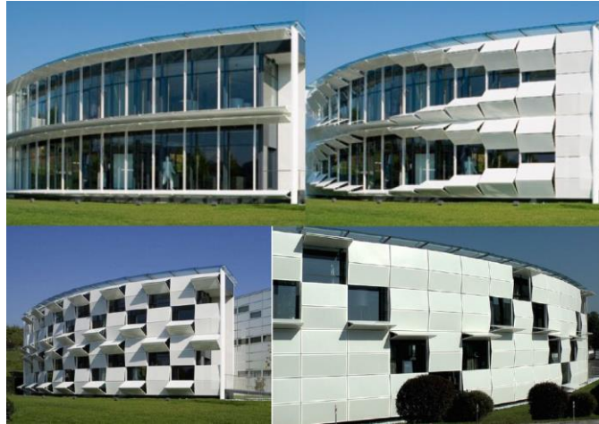
b) Shadowing: The dynamic façade of the Kiefer technical showroom
