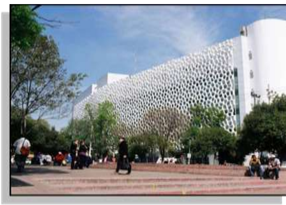
Picture showing Torre de Especialidades hospital building in New Mexico
