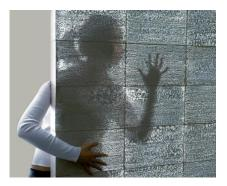
Figure 17 Translucent Concrete partition
